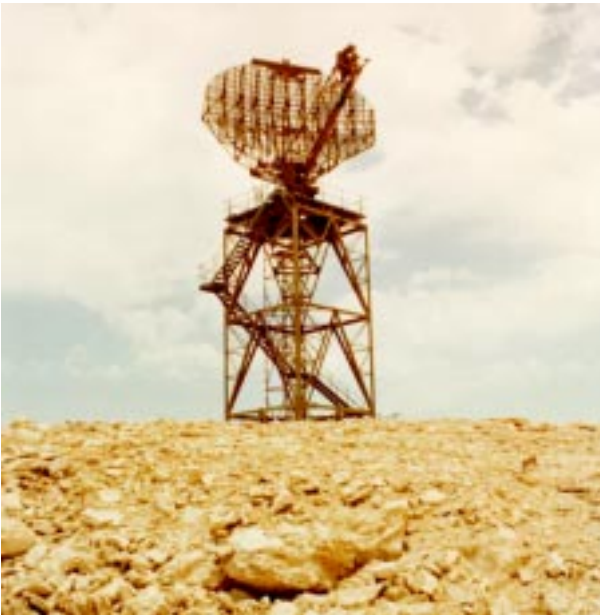
17 Typical air traffic control radar in a desert environment
